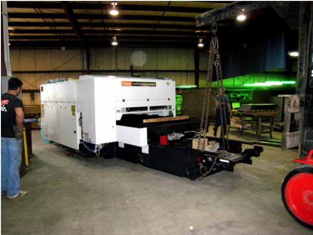
The new unit is moved into position, and being prepped for final installation.
